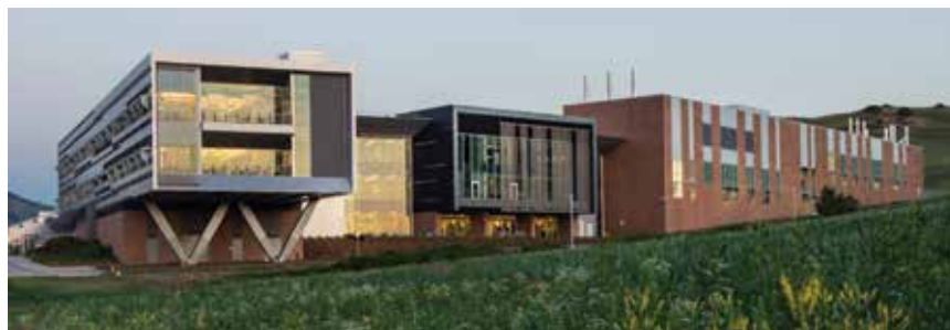
The high performance precast concrete enclosure had an effective R-value of R-28.4. Photo: Dennis Schroeder, NREL.
